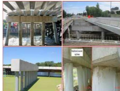
**Figure 1:** Pile Caps Behave as Continuous Deep Beams
